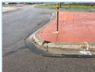
Curb and Gutter
