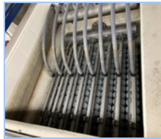
Membrane Replacement Pic
