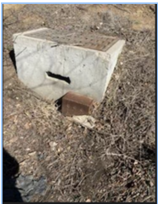
Storm Structure Rehab 5
