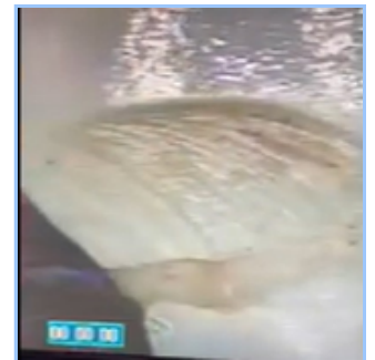
Ripple-fold in liner
