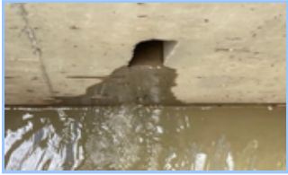
Storm Structure Rehab 1
