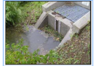
Storm Structure Rehab 4
