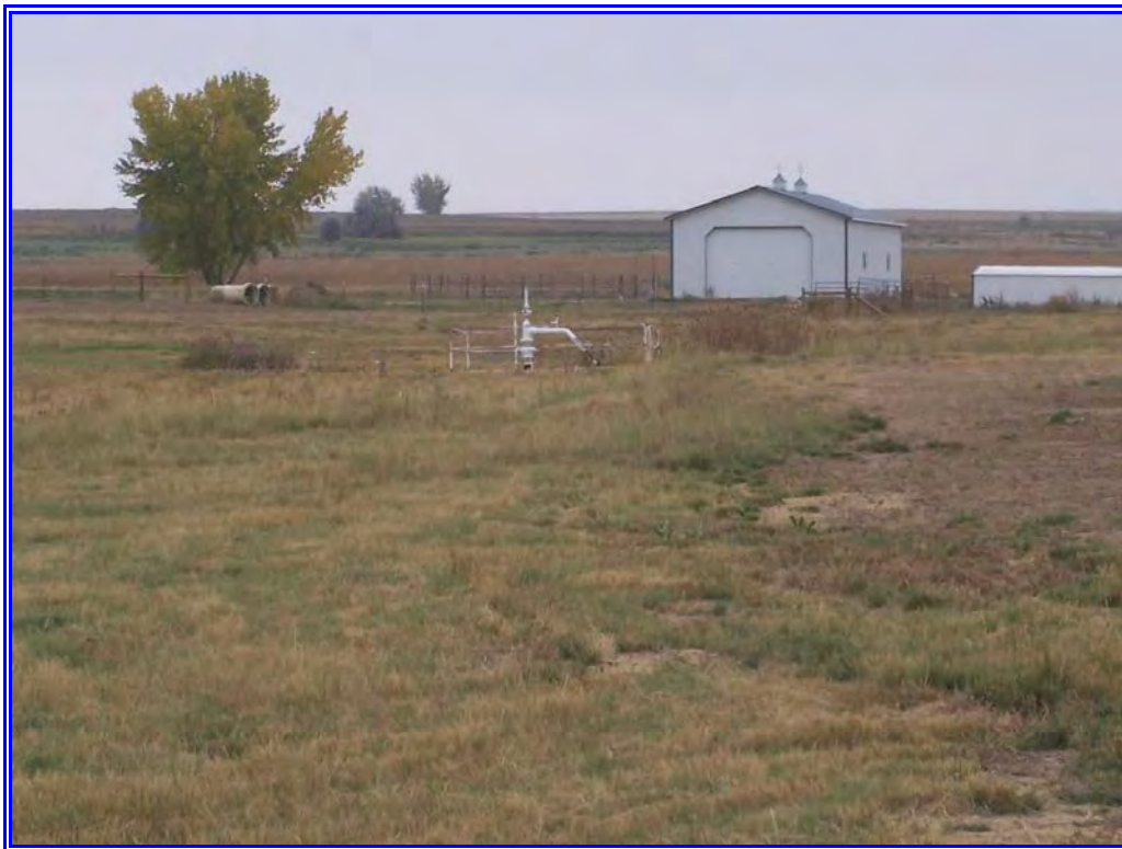
Leased equipment shed northwest portion of site
