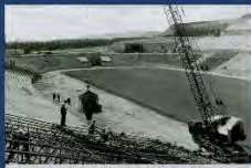
Elliptical shape of the stadium required the invention of a traveling form to pour concrete for the stands. (1962)
