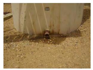
**Photo #19** – View of the stained soil beneath the eastern most oil and/or natural gas AST.
