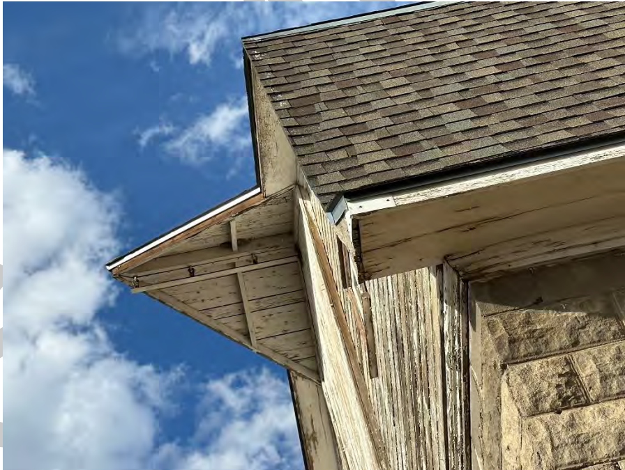
Figure 10: Detail view of roof and eave conditions.
