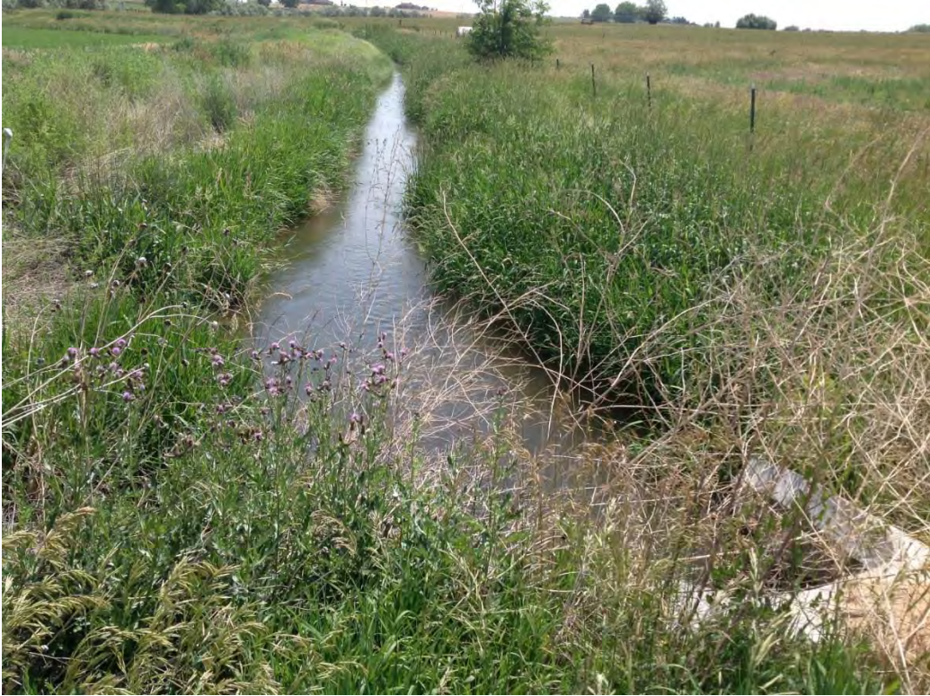
Overview of 5WL5461.3 showing large modern concrete culvert, facing east.
