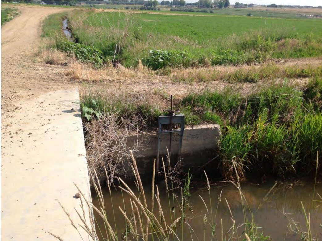
Overview of 5WL2248.14 Feature 4 headgate, facing north.
