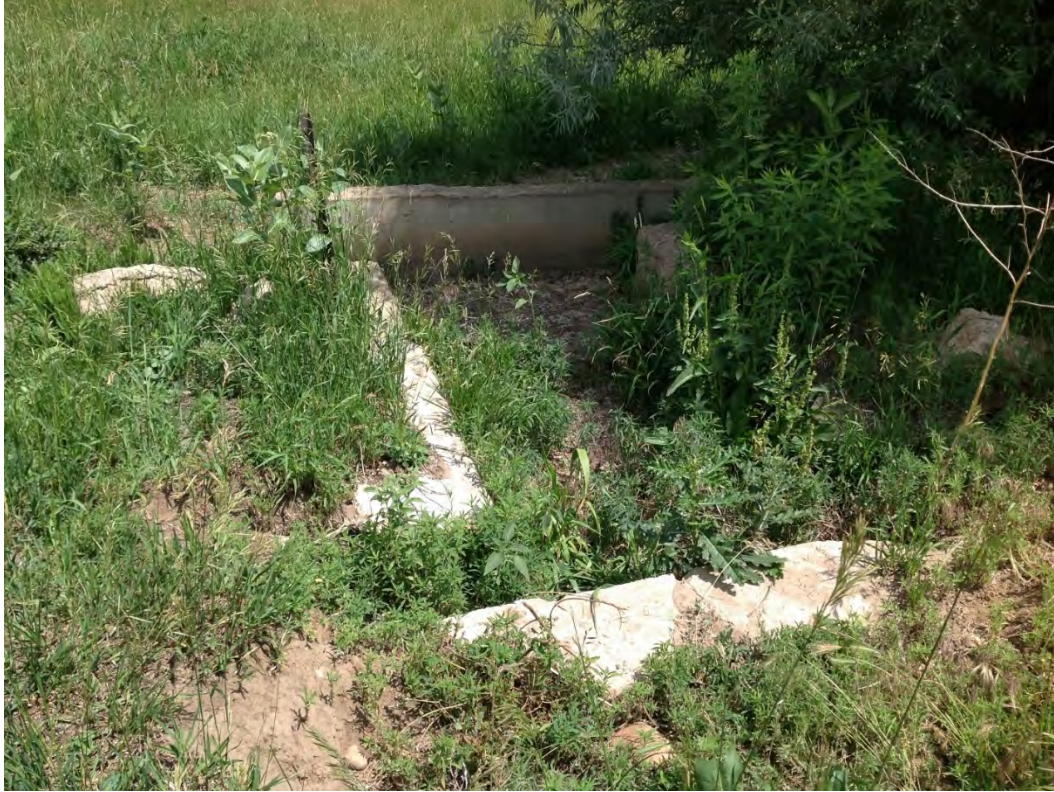
5WL1526.4 Feature 1, facing north.
