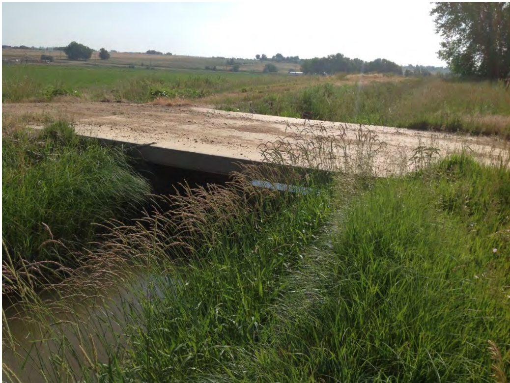
Cement bridge across 5WL2248.14 for dirt access road, facing east.
