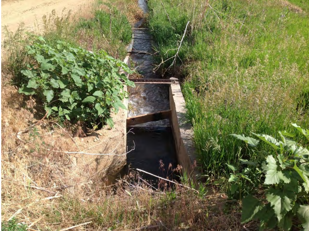
Overview of 5WL2248.14 Feature 4 drop complex, facing north.
