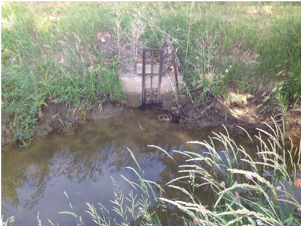
Overview of 5WL2248.14 Feature 1 facing west.
