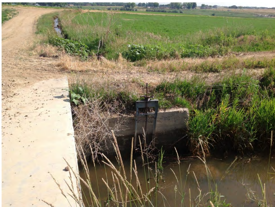
Overview of 5WL2248.14 Feature 4 headgate, facing north.
