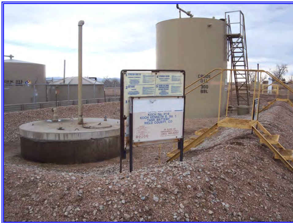
One of the 28 petroleum production facilities on the project
