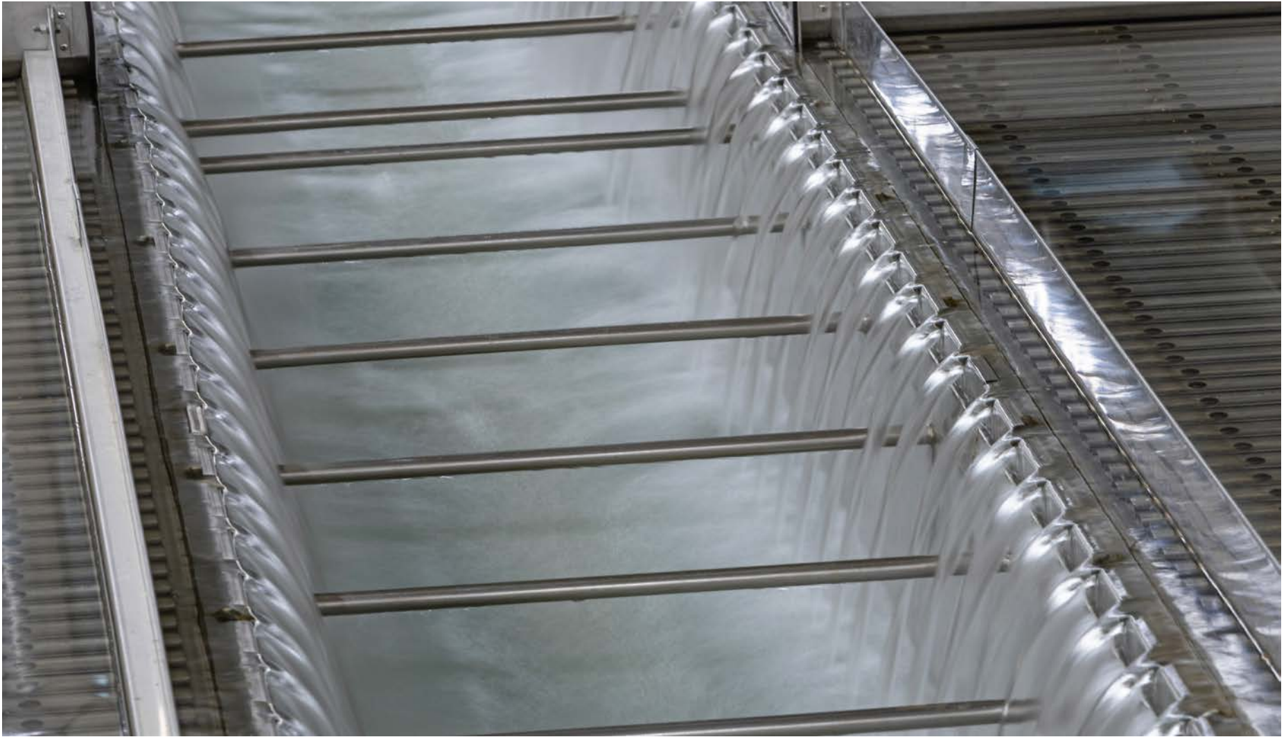
Sedimentation Basin (clarifier), Weir and Launder (a type of aqueduct!)
