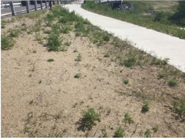
Figure 1. Soil surface conditions observed on the south side of Erie Parkway. This material will need to be removed to ensure successful germination.
