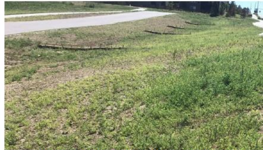
Figure 4. Straw wattles with sediment build up on the upslope position at each placement.
