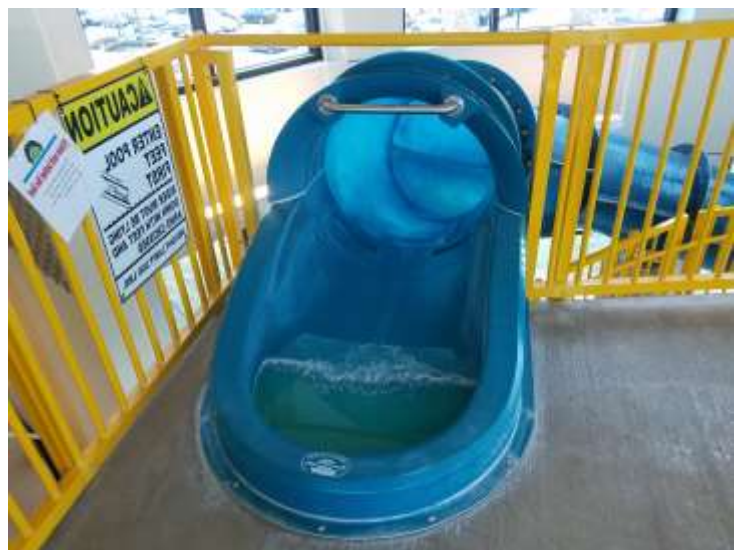
Gel Coat Interior and Paint Exterior of (1) Enclosed Waterslide
