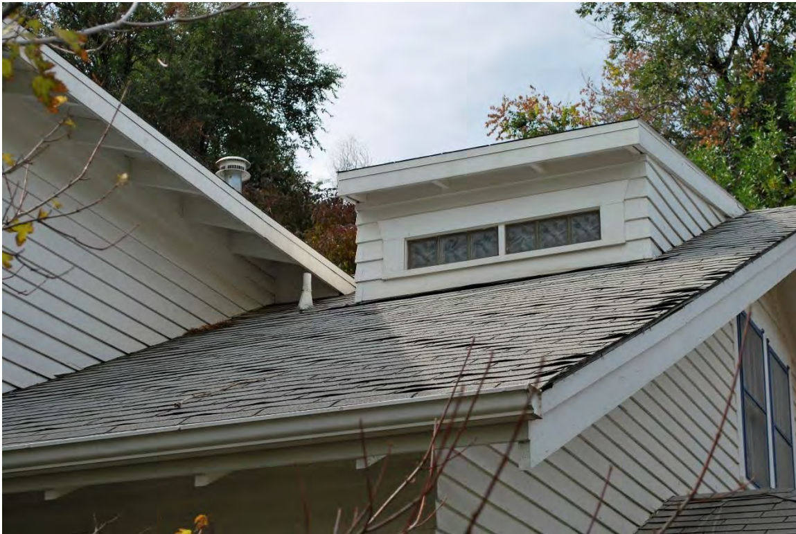
Oct. 9, 2015, Image 12: Detail of Contemporary Shed Dormer
