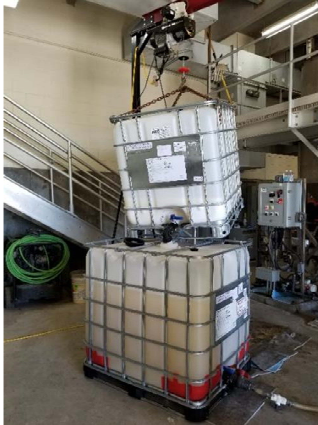
Figure 7-9 Existing Dewatering Polymer Transfer System
