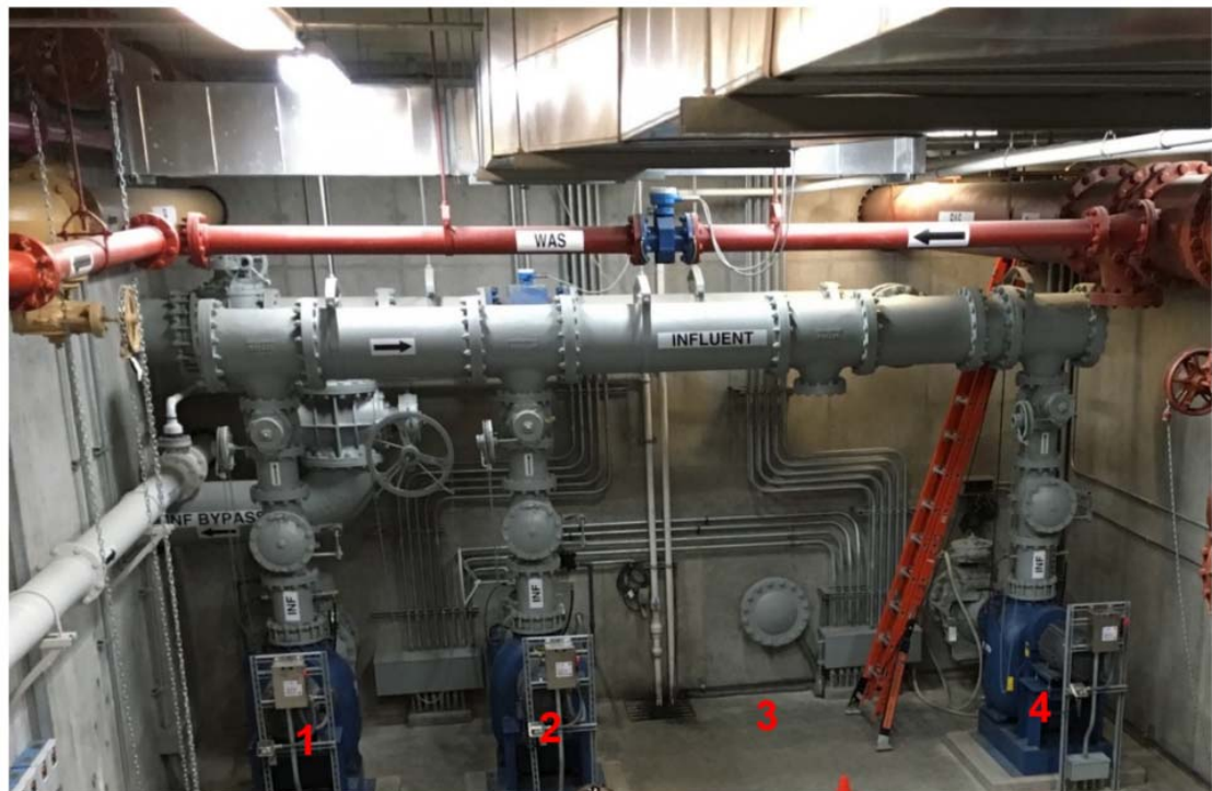
Figure 5-5: Erie NWRF Influent Pumping
