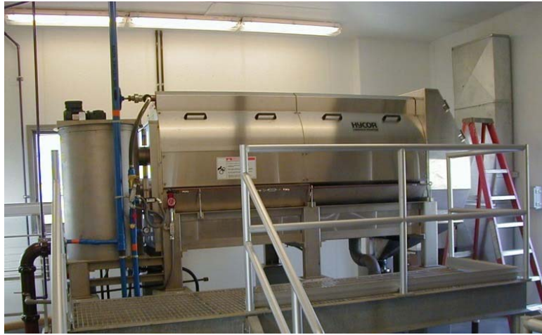
Figure 6-26. Parkson Hycor Rotary Drum Thickener
