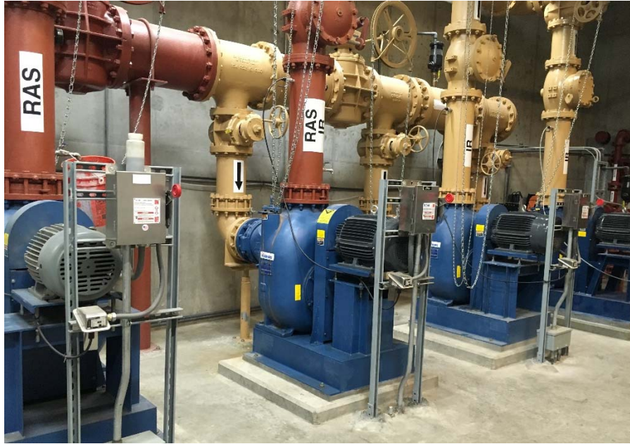
Figure 5-12: NWRF RAS/IR Pumping
