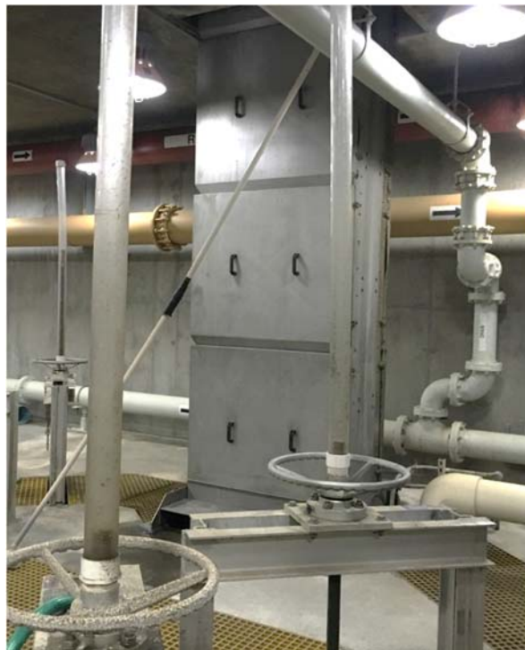
Figure 5-4: Erie NWRF Headworks Screen
