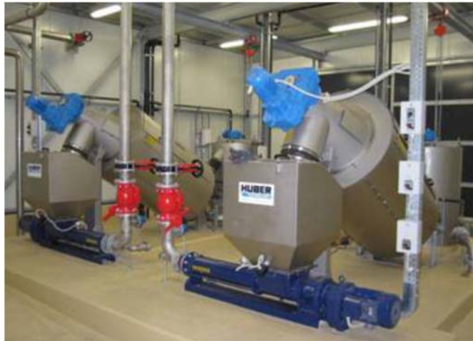
Figure 6-27. Huber Screw Press Thickener
