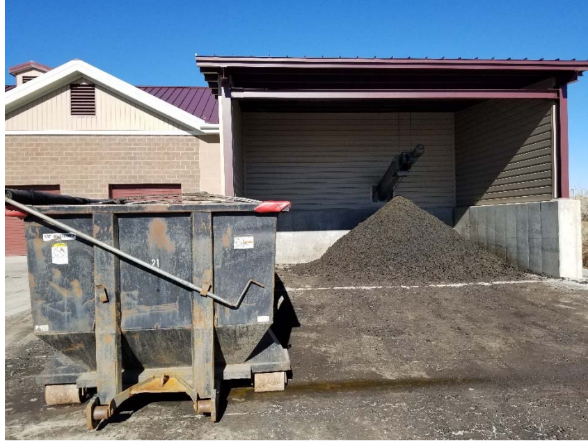
Figure 6-10: NWRF Conveyance and Loadout System
