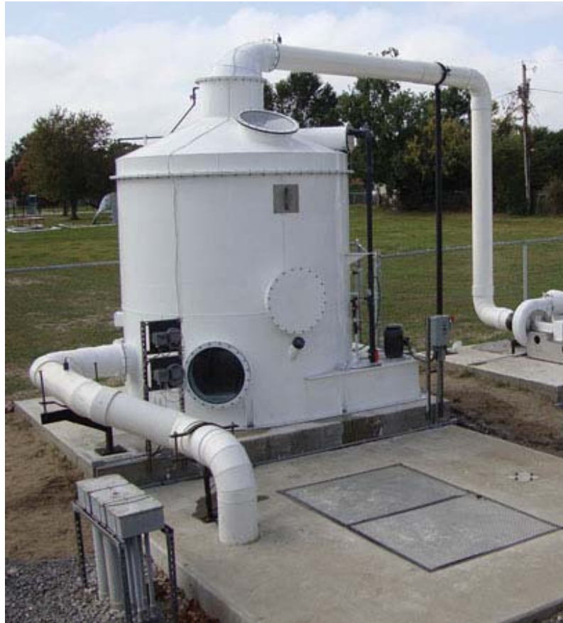
Figure 7-3. Example Biotrickling Filter System
