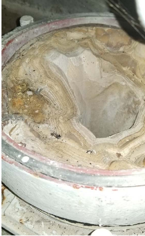
Figure 6-9: NWRf Pressate Return Piping Mineral Build-up
