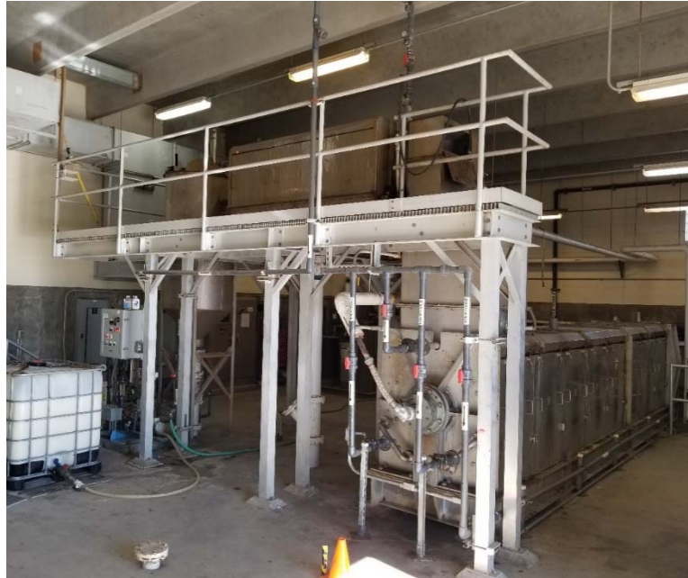
Figure 6-8: NWRf FKC Dewatering Screw Press
