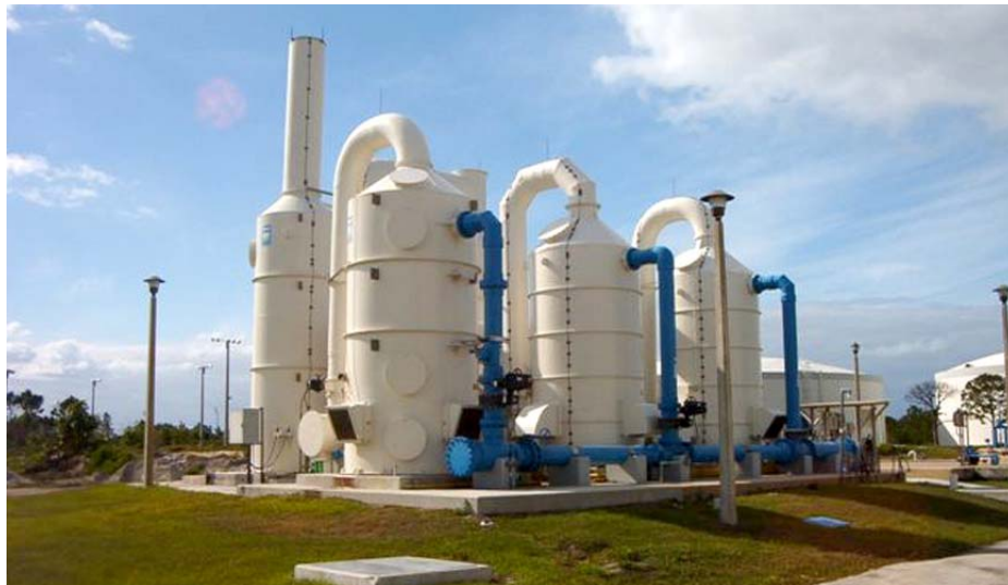
Figure 7-5. Example Chemical Scrubber System
