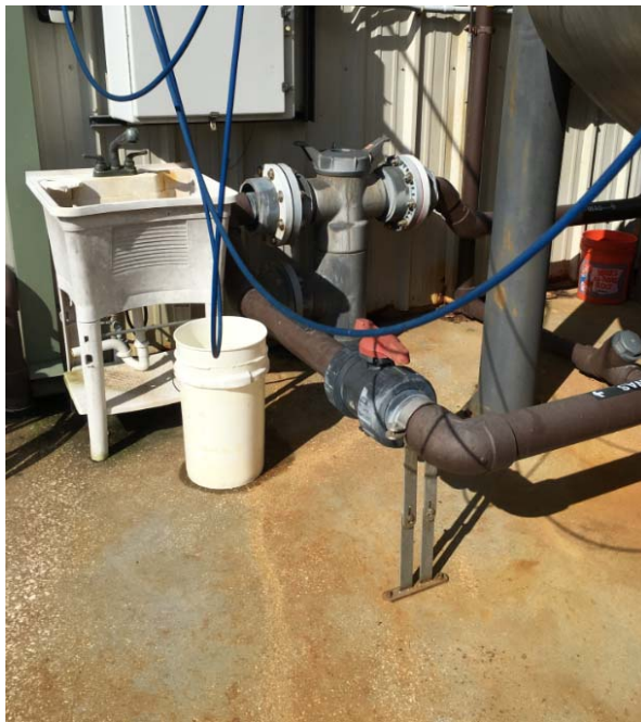
Figure 6-17: Increased Concrete Corrosion at Neutralizer Installation
