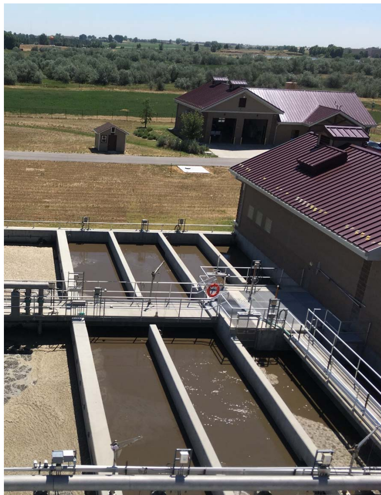
Figure 5-6: Erie NWRf IFAS and Grit System
