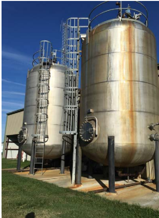
Figure 6-16: BCR Neutralizer System
