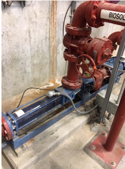
Figure 6-5: NWRF Solids Dewatering Pumping
