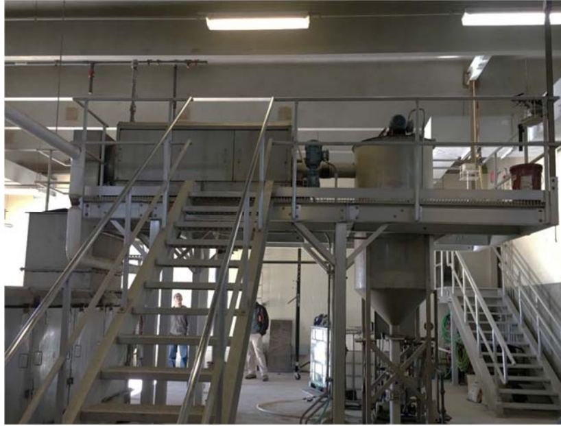
Figure 6-7: NWRf WAS Thickening System
