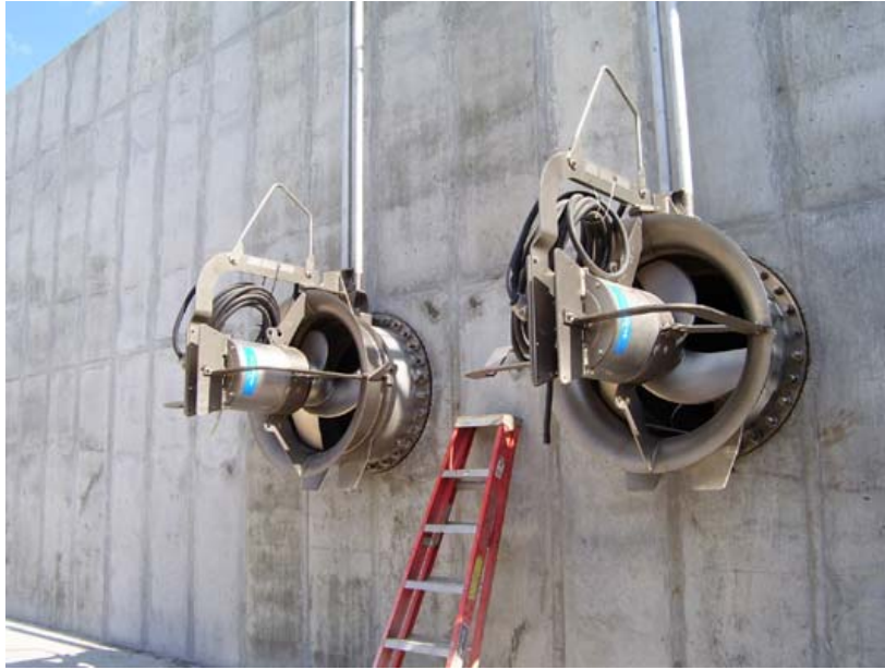
Figure 5-13: Propeller Style In-Basin Pumps Example
