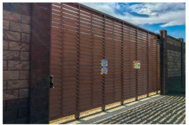
MATERIAL: WEATHERING (COR-TEN) STEEL OR ALUMINUM COLOR: NATURAL PATINA OR POWDER COAT COLOR TO MATCH WEATHERING STEEL NATURAL PATINA
