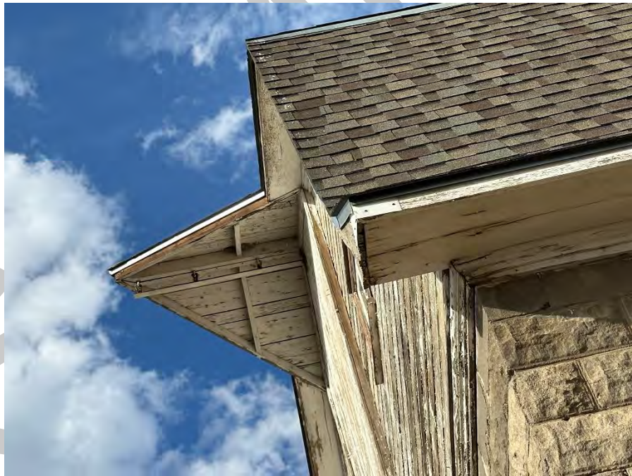
Figure 10: Detail view of roof and eave conditions.
