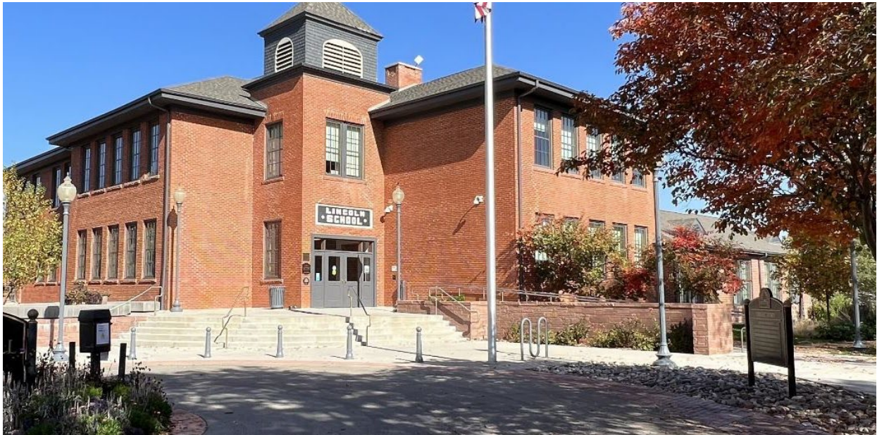
Photo 2: Current state of the bell tower. Louvres were added in a past renovation.
