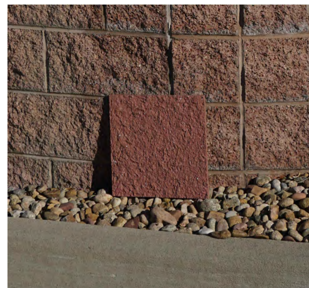
(PROPOSED) FRP STUCCO, COLOR TO MATCH EXISTING DARK COLORED CMU: STEALTH - TEXTURED BLOCK FRP SAMPLE 6053 SUPERPAINT (B30FXR9666) SAMPLE 3A
