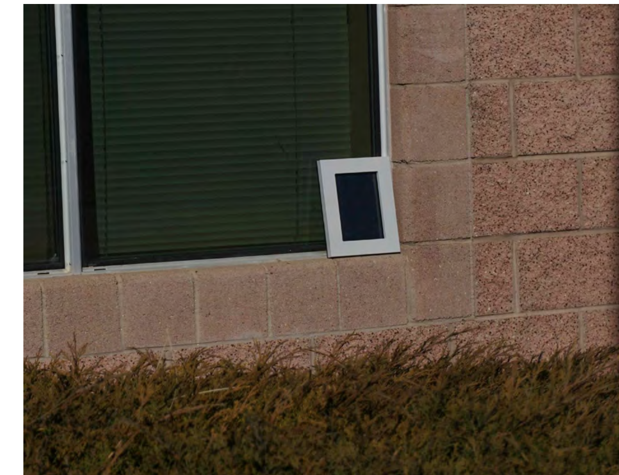
(PROPOSED) FAUX WINDOW TO MATCH EXISTING: 40 / 30 STEALTH CORE PANEL CLEAR ACRYLIC 6858 COROTHANE SATIN / FRP SAMPLE 2A
