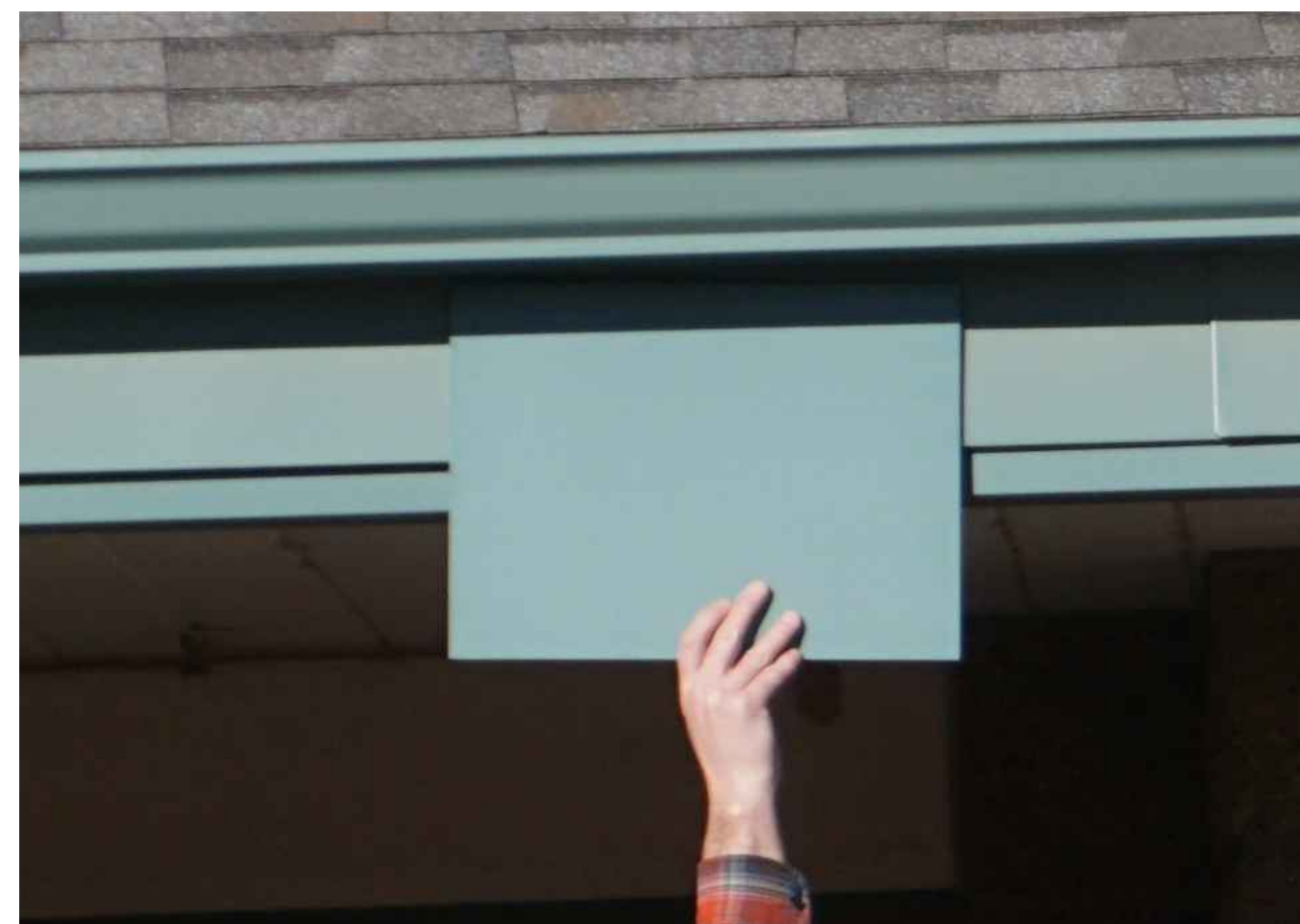
(PROPOSED) FRP TO MATCH (E) FASCIA: STEALTH - SMOOTH FRP SAMPLE 0047 COROTHANE FLAT (B65XXL12698) SAMPLE 4A
