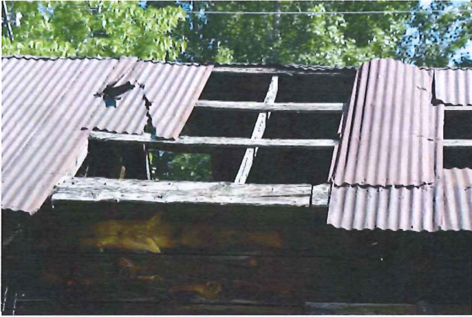
Site 5: Granary: Roof Detail
