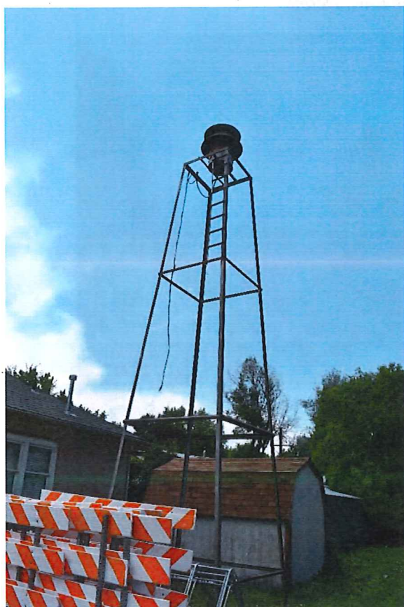
City Hall: Siren Tower at North Elevation
