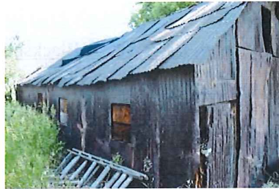
Site No. 2: Blacksmith Shop
