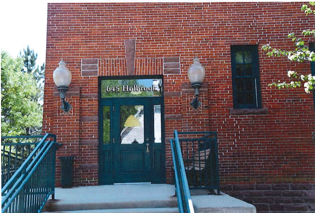
Lincoln School: North End of West Elevation
