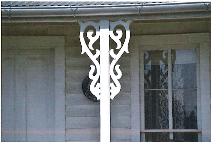
Site 6: Farm House: Porch Bracket Detail
