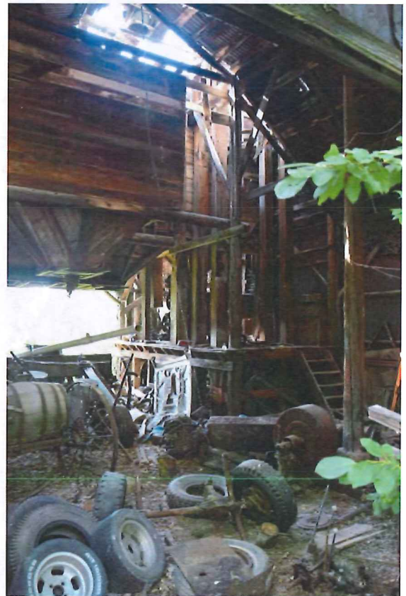
Site 3: Mill: Interior
