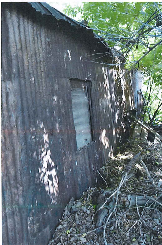
Site 2: Blacksmith Shop: East Wall
