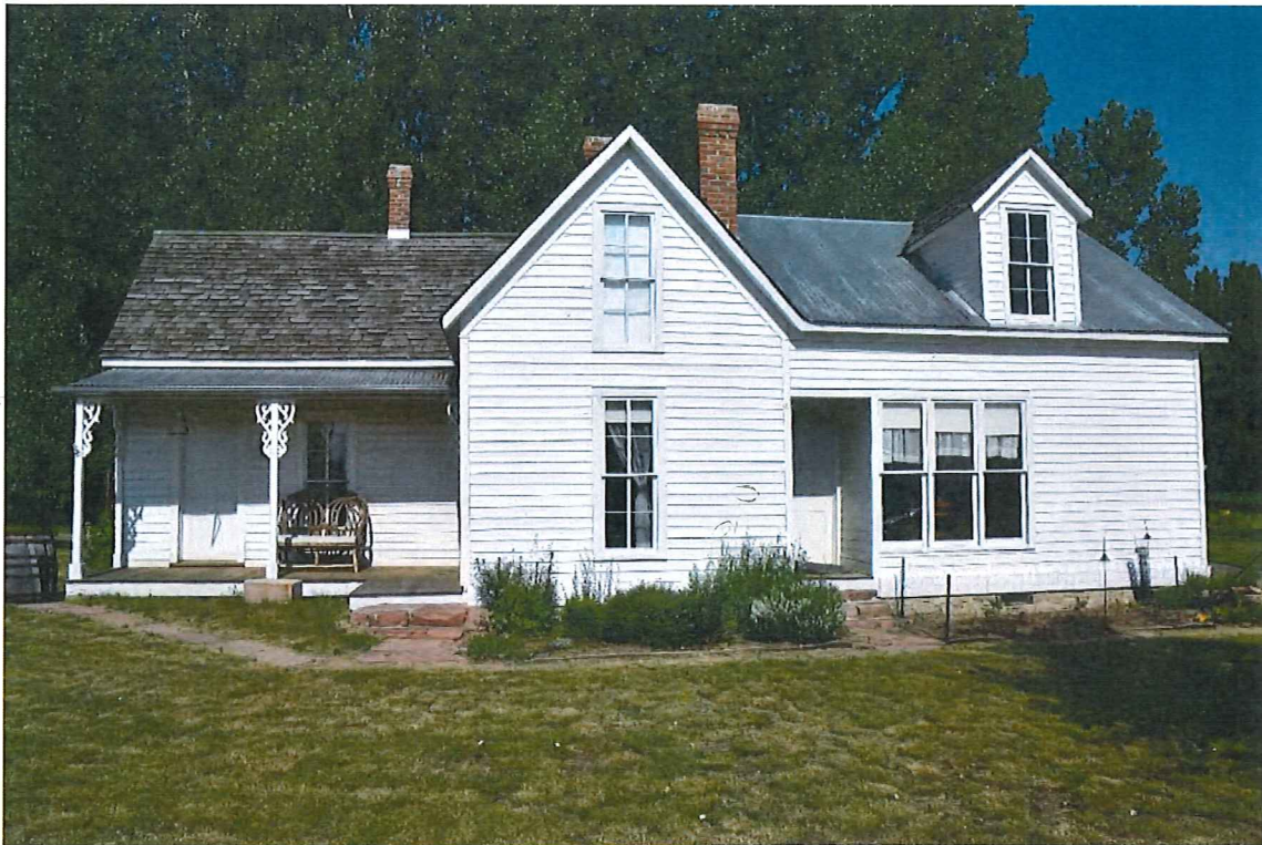
Site 6: Farm House: East Elevation
