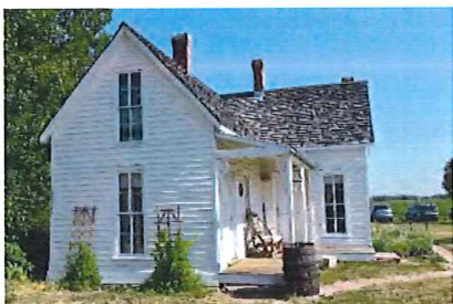
Site No. 6 Farm House
