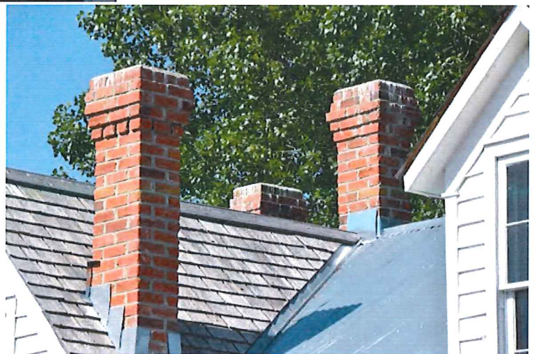
Site 6: Farm House: Roof Detail
