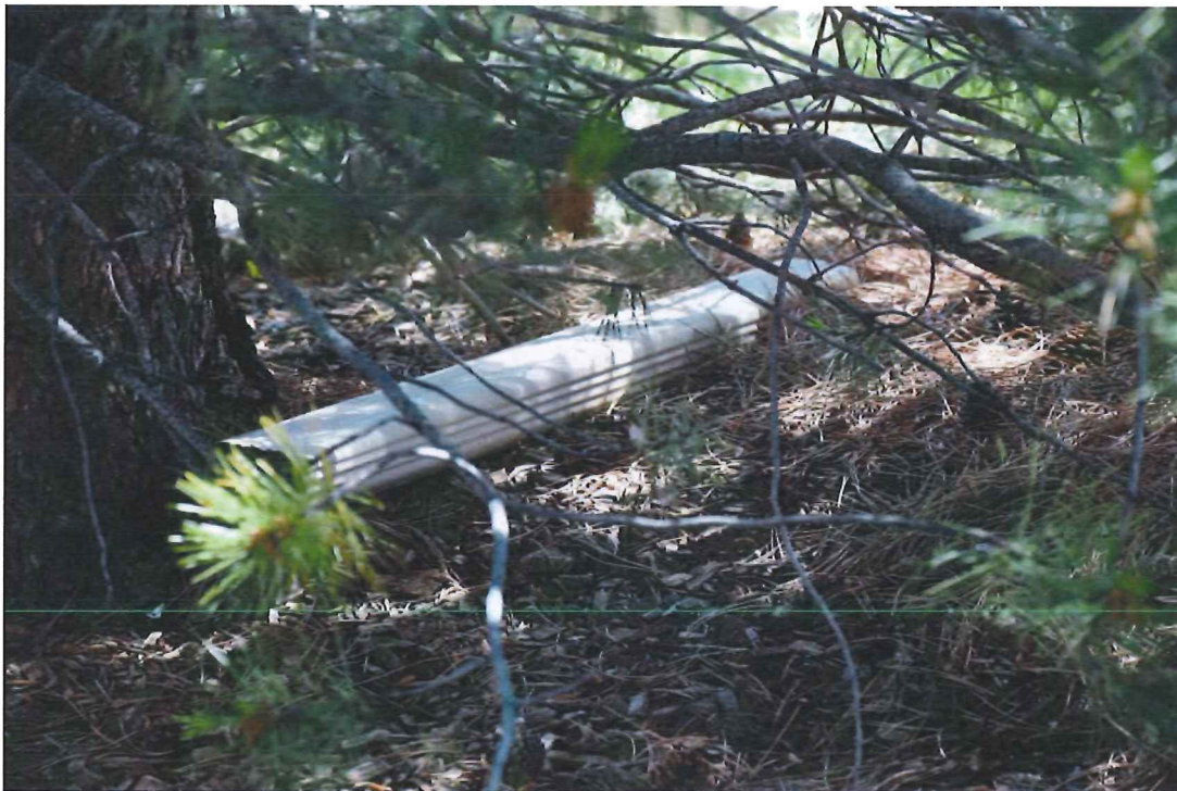
Lincoln School: Downspout Extension Under Nearby Tree
