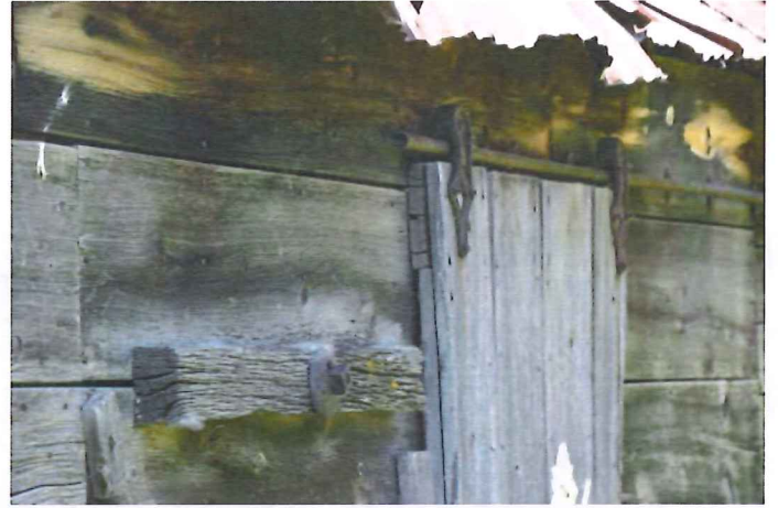
Site 5: Granary: North Wall Detail
