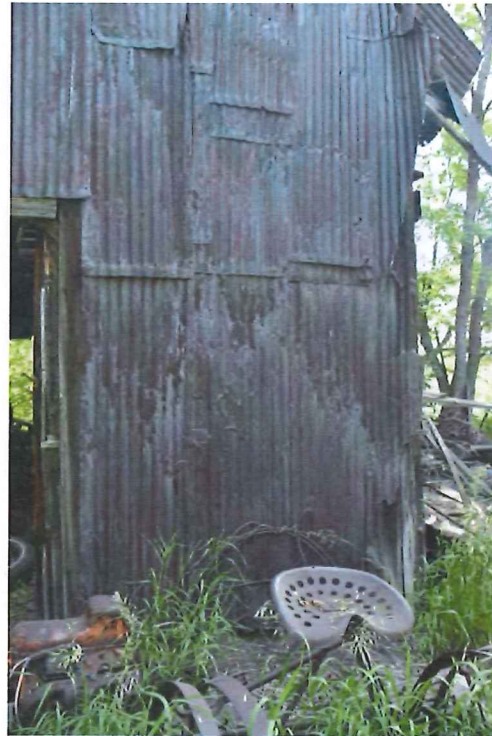
Site 3: Mill: West Wall
