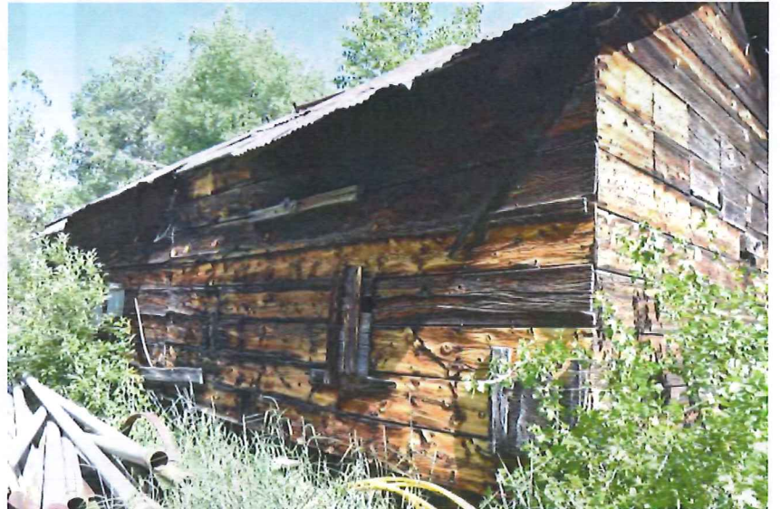
Site 5: Granary: Southeast Corner
