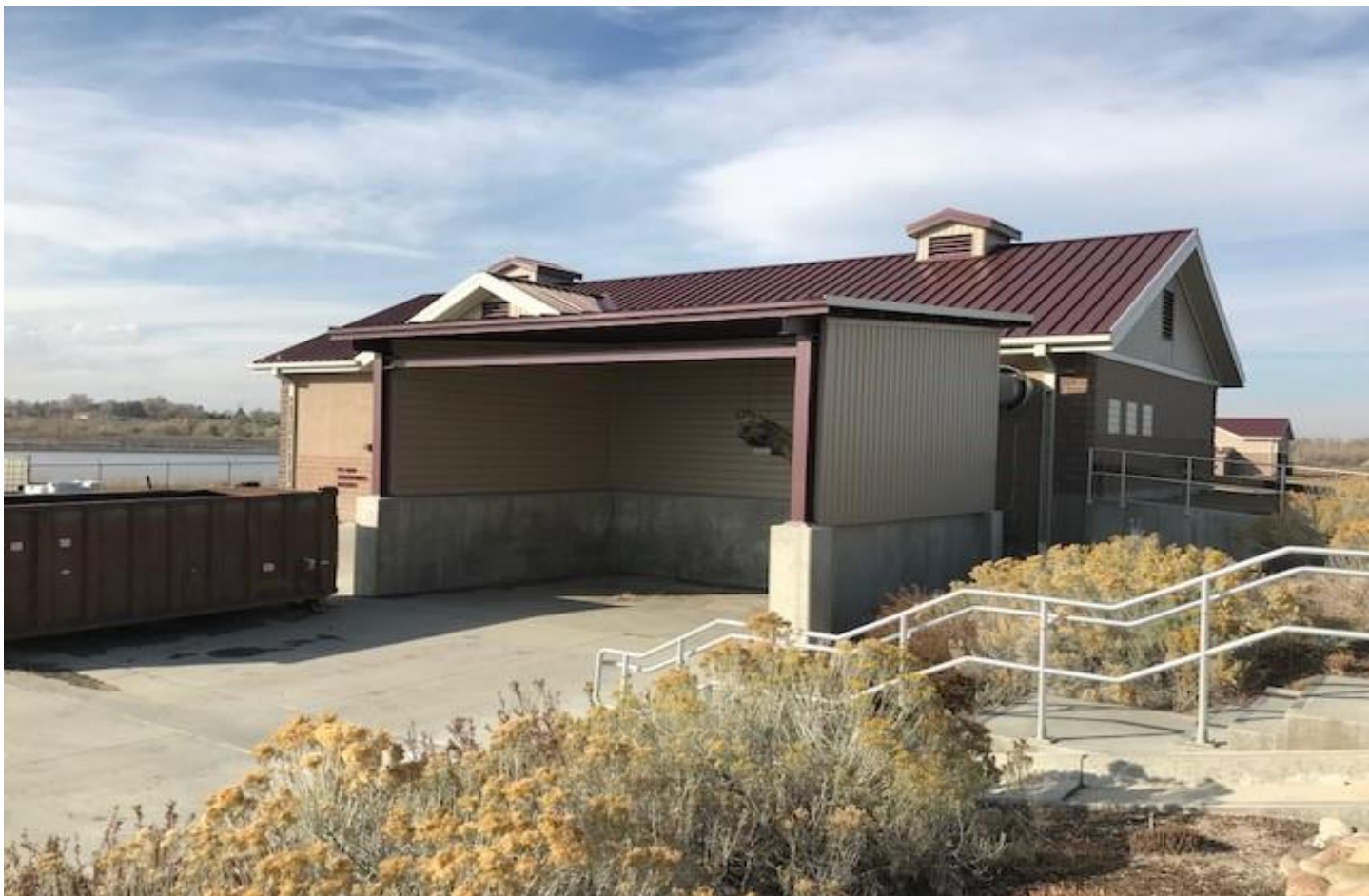
Odor Reducing Enclosure at Solids Handling
