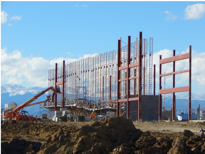
Figure 9: Commercial building construction in Erie.
