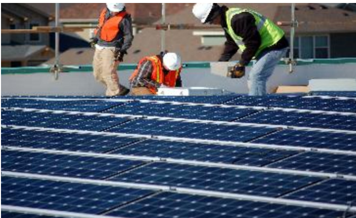
Figure 4: Solar panels being installed at the Leon A. Wurl Service Center.
