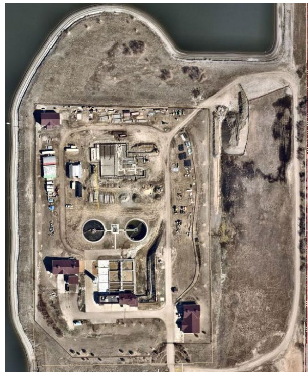
Erie’s Wastewater Reclamation Facility
