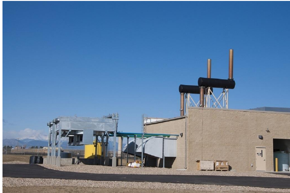
Methane Recovery Facility at FRL
