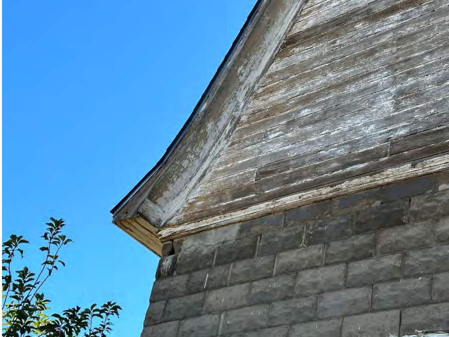
Figure 7: Masonry, trim, and eave conditions at the west gable end.
