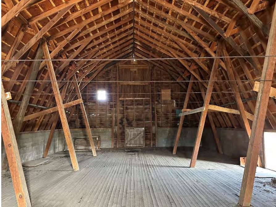
Figure 11: Overall view of second floor hayloft space. Note that exterior insulation is proposed at the roof and gable ends to maintain the historic character and appearance of this unique space (interior work not in scope).
