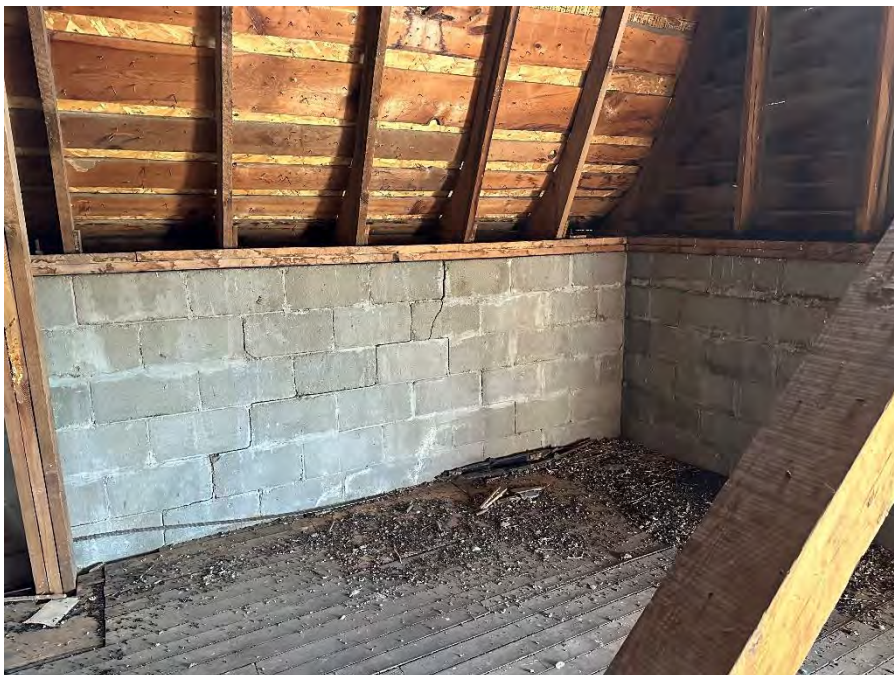
Figure 12: Cracks visible at concrete block on the second floor of the building. Note that some of the cracks visible on the exterior telegraph through to the interior (interior not in scope).
