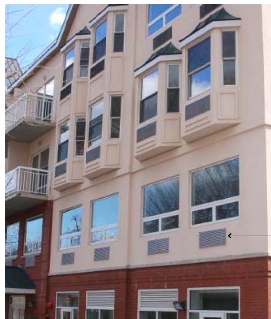
EXAMPLE - PACKAGED TERMINAL GAS HEAT & AC UNIT (can be added as required)
