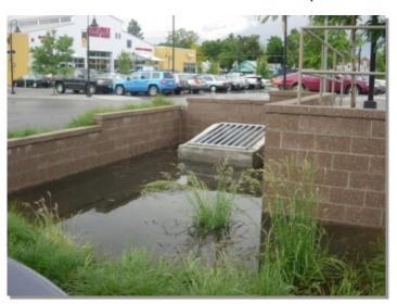
**Photograph EDB-3**. Although walls may complicate maintenance access, this outlet structure is relatively hidden from public view. This photo was taken shortly following a storm event.
