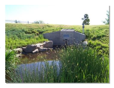
**Photograph EDB-2**. The initial surcharge volume of this EDB is contained within the boulders that surround the micropool.
