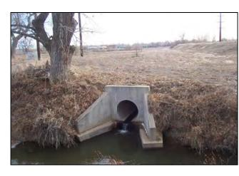
The Old Town outfall is primarily located in the Town of Erie. A small area of unincorporated Weld County is located near the outfall at Coal Creek. The outfall is comprised of a series of storm sewer pipes that convey stormwater runoff to Coal Creek.
