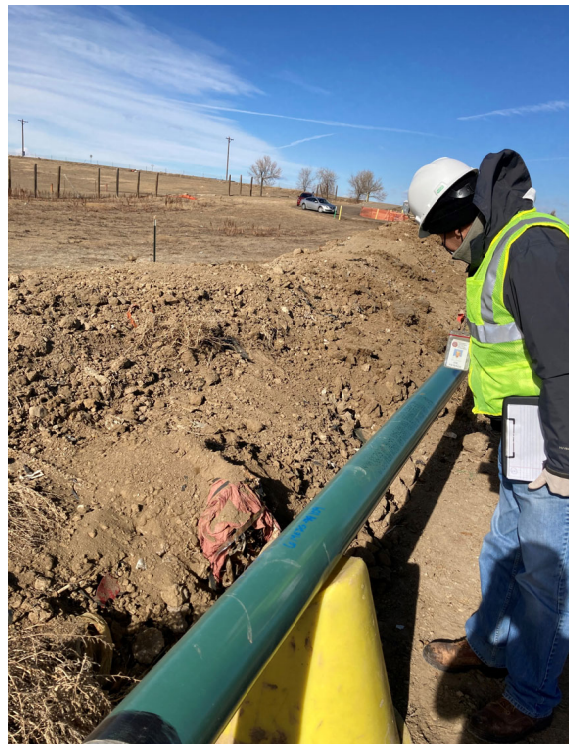
CDPHE Inspector @ WM Site
