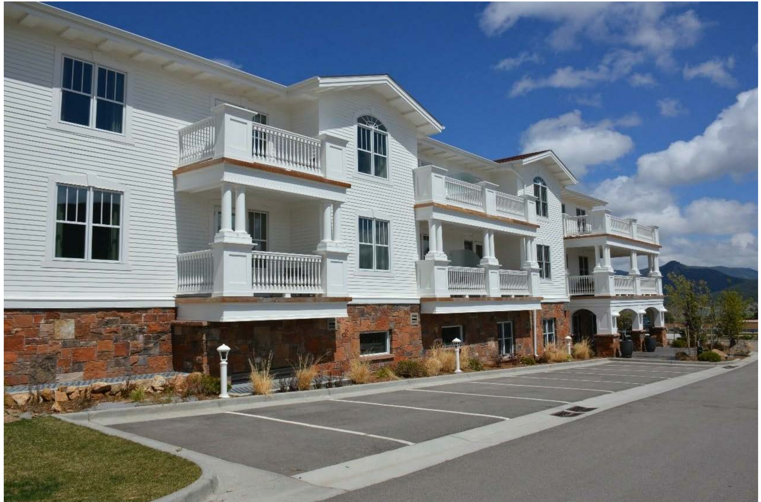
GEORGIAN MIXED-USE COMMERCIAL - THE STANLEY HOTEL ASPIRE HOTEL CENTER, ESTES PARK, CO
