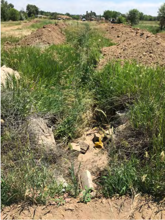
Photo 12 – Photo taken on the west side of Filing No. 8, at west end of irrigation lateral #4, facing east. Oil and gas pad is visible in the distance. Note lack of wetland vegetation in the ditch and piles on new fill dirt along each side of the ditch.
