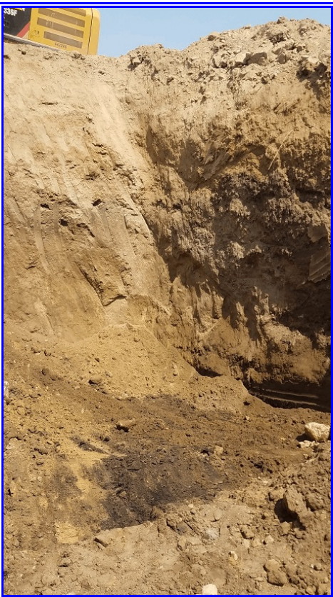
Base of excavation showing shaft outline
