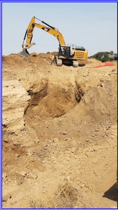
Excavation for Chase Mine Shaft
