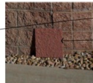
(PROPOSED) FRP STUCCO, COLOR TO MATCH EXISTING DARK COLORED CMU: STEALTH - TEXTURED BLOCK FRP SAMPLE 6053 SUPERPAINT (B30FXR96 66) SAMPLE 3A
