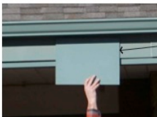
(PROPOSED) FRP TO MATCH (E) FASCIA: STEALTH - SMOOTH FRP SAMPLE 0047 CORDTHANE FLAT (B65XXL126 98) SAMPLE 4A
