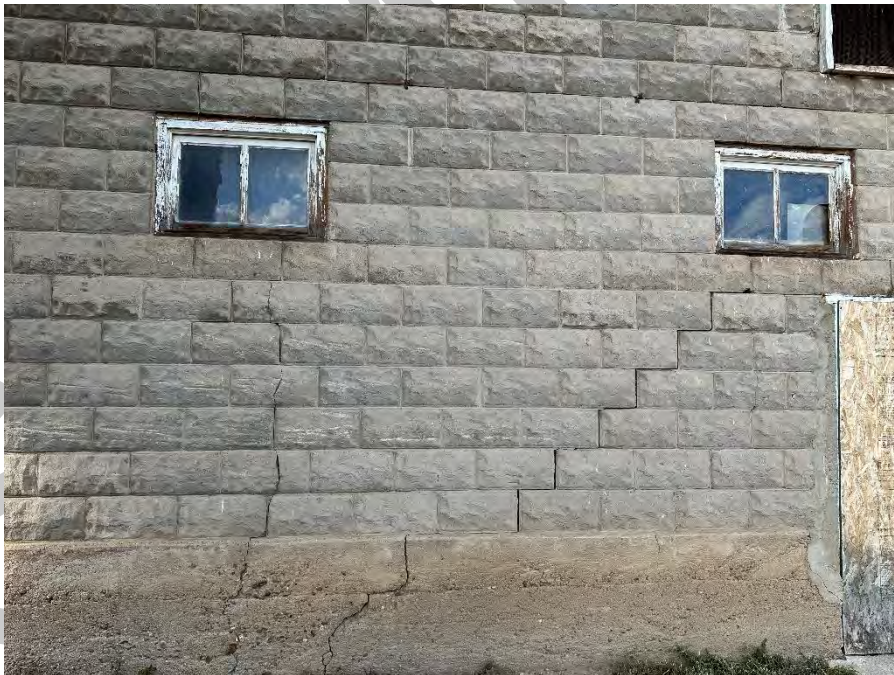
Figure 8: Detail view of exterior window and masonry conditions. Note deterioration of original wood windows and cracks visible in the concrete block masonry.
