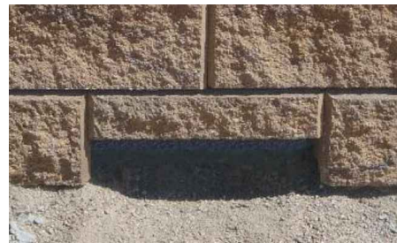
OPENING FOR WATER DRAINAGE
