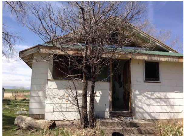
Photo 2. View west at tree 5. Growth is constricted by proximity to house.
