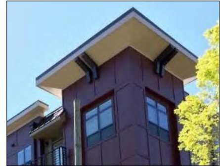
Figure 75 - Example of a large eave overhang.
