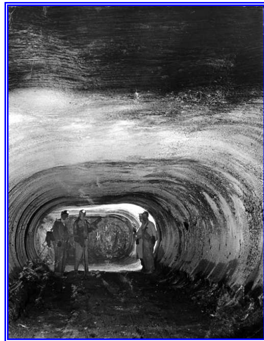
Photo of Room Mined Using Continuous Miner
