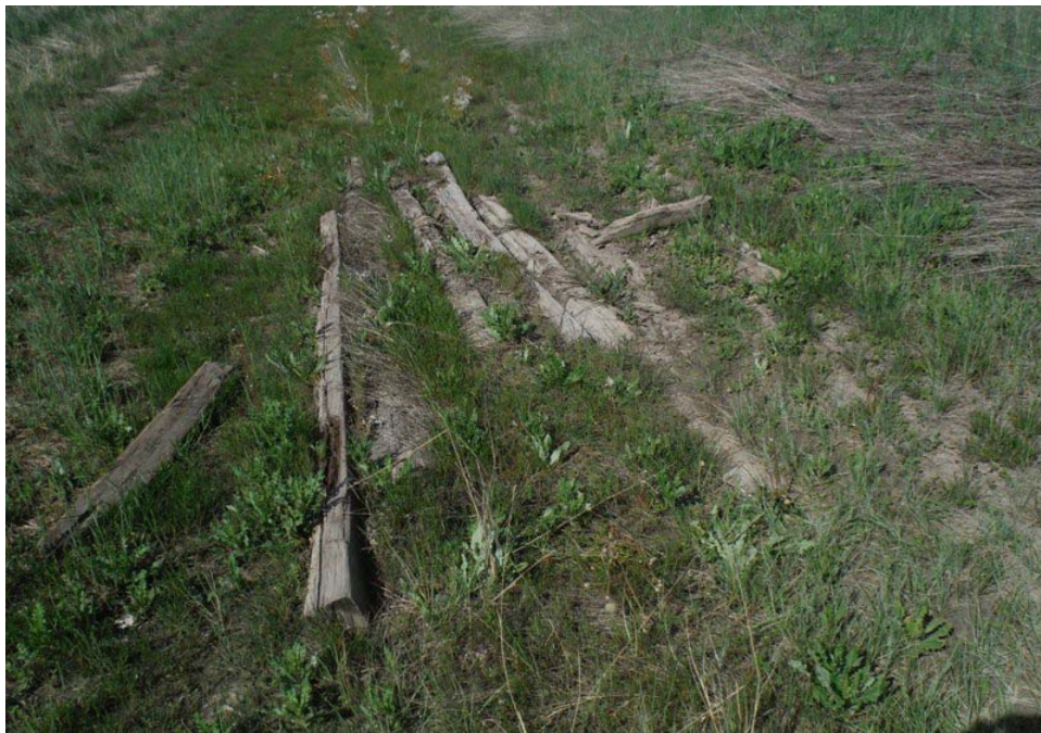
5WL1423.44, western portion of railroad segment. View to the west of wood poles and a railway tie associated with the railroad berm.
