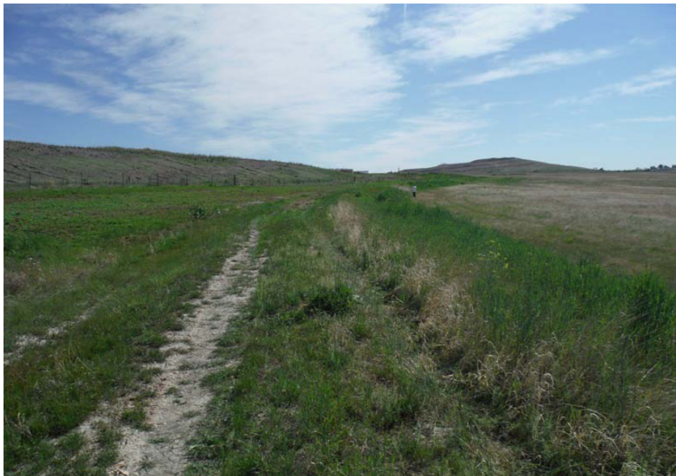
5WL1423.44, western portion of railroad segment. View to the east showing the railroad berm and the existing two-track road on top of it.
