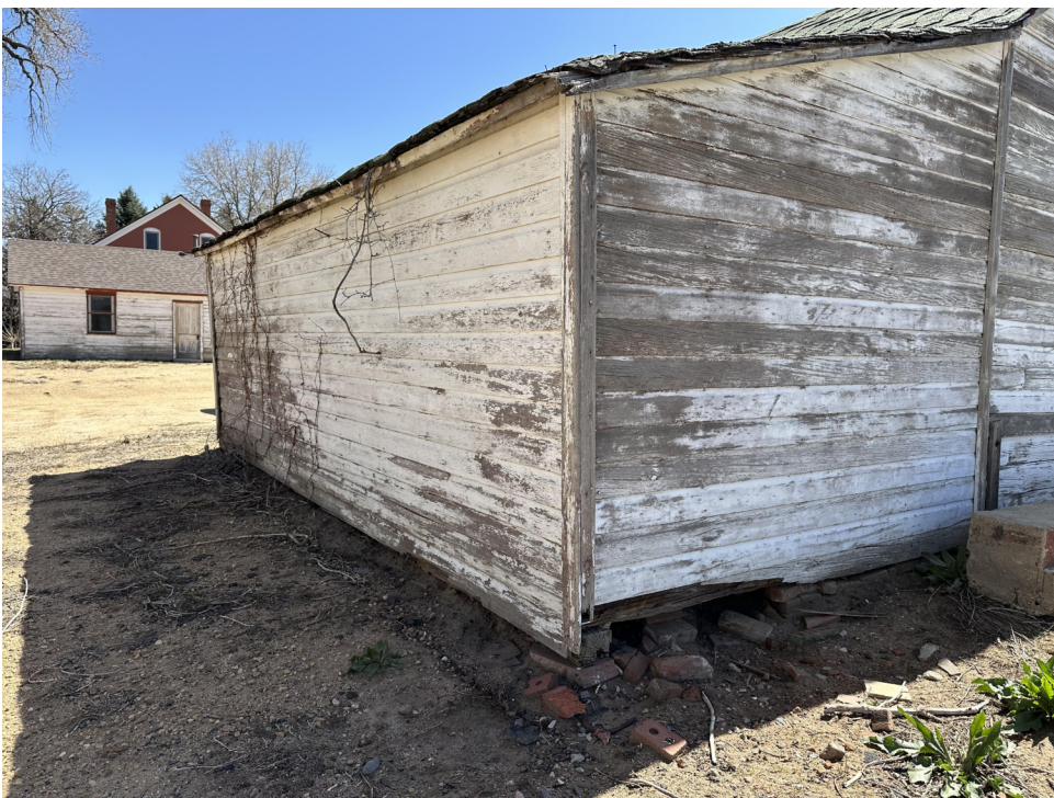
EXISTING BARN SIDING PHOTO
